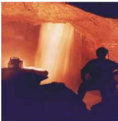
Such incident can be avoided by doing pre-injection in tunnel using appropriate Polyurethane or other injection grouting system. Pre injection is always safe and less costly and can be planned and done in advance if One has prior information on the presence of water bound strata along the tunnel axis of excavation.
